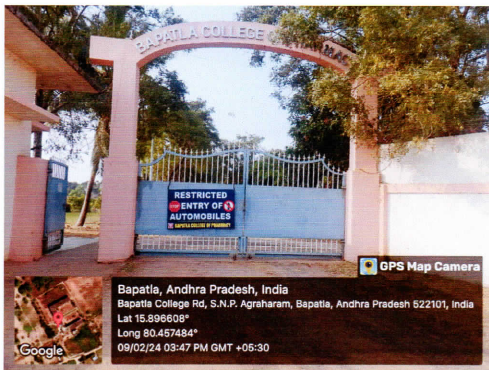
No entry of automobiles Caution Board
